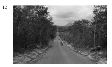
This photograph shows a good gravel road. It has a camber, side drains and mitre drains, although the latter are hard to see. With two or three years of vegetation growth on the shoulders and side slopes, the road will be more durable and erosion resistant.
