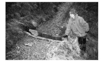
This narrow stone lined channel allows pedestrians to cross a stream with ease and prevents erosion of the footpath. It is a very low cost improvement. If the hillside below the path were prone to erosion, an outfall structure would be required. The channel can also collect and dispose of water that might flow down the footpath itself.
