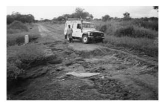
It is important to correctly determine the flow requirement of a culvert. This single aperture culvert was built without consideration of the catchment area and potential run off volume. In a single storm it overtopped and rendered the road accessible to only four wheel drive vehicles.
