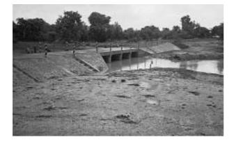
In many situations, a road may cross a water course and then continue across low lying land. An isolated bridge would cross the water course, but embankments are needed to provide access along the entire route. This photograph shows a submersible bridge between embankments that will provide year round access.
