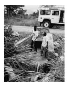
Erosion began in this culvert outfall channel some distance downstream. The erosion has moved upstream and is now undercutting the apron, putting the entire structure at risk of collapse. Run-off around the wingwalls has contributed to the problem. The downstream erosion needs to be controlled by reforming the channel and constructing scour checks. Then any structural damage should be repaired, and the wingwalls extended down to apron level and backfilled.
