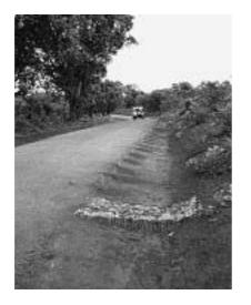
This photograph, looking downhill, shows a scour check to reduce erosion. It is well built with wooden stakes and stones and well shaped to keep the water flowing in the centre of the drain. A mitre drain was dug at the bend in the road but more should have been dug to divert the water onto the surrounding land. Grass has also been planted along the shoulder line in an attempt to prevent erosion.
