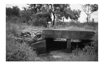
This culvert is free flowing and the road is currently passable, but the outfall channel is blocked with silt and high vegetation. An inadequate attempt at repairing the erosion behind the wingwall will put access at risk in the likely event of further overtopping. The erosion should be properly repaired and the outfall channel fully cleared.
