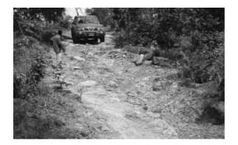
Four wheel drive passage down this extremely rocky track is very slow and requires great care, while the vehicle, particularly the tyres, can be damaged. This track is clearly not providing safe and reliable access. Providing access will require major improvement work or route realignment.
