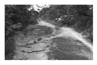
Rain falling on the surface of this inclined track flows down the gradient forming small erosion channels. Little water absorbs into the well compacted fine soil. The channels concentrate the water and can grow into severe longitudinal erosion. The track has become impassable and vehicles must detour through the undergrowth. The track should be reformed with camber, side drains and mitre drains or the solution shown below can be used.
