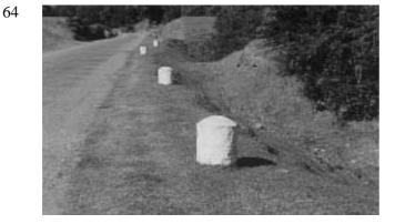
This photograph shows low cost edge delineators being used to indicate a steep drop. They are made from half-buried oil drums filled with sand and capped with concrete. They are painted white for greater visibility, particularly at night.
