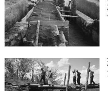
This double culvert has masonry walls upon which a reinforced concrete cover slab is being built. Previously excavated soil is used as formwork for the cover slab and will be removed when the concrete has gained sufficient strength.
