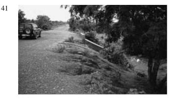
This road shoulder is badly eroded. The extent of erosion can be seen from the height of the wingwall, originally at ground level. Shoulder erosion often occurs near water crossings as water concentrates at the low point on the road surface and then runs off the shoulder. The shoulder should be reconstructed and vegetation planted on the steep slope.
