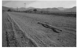
This road has corrugations approximately 75 mm deep. Access has not been lost and vehicle operating costs (VOCs) are not high, but the road is dangerous to travel on at speed as control can be easily lost. Dragging can eliminate initial minor corrugations and prevent the problem getting worse, but grading is required when they reach this advanced state. (Photograph courtesy of CSIR, South Africa)
