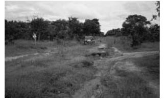
Run off from the surrounding land is causing serious erosion to this very badly maintained road. It is necessary to protect the inside face of the side drain or to dig interception drains to channel the water to a water course or a culvert. Interception ditches are more effective than drain lining, but maintenance can often be overlooked if they are out of sight.
