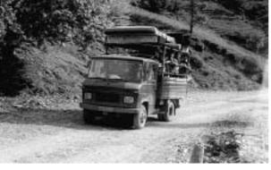
A stone surface remains passable for many years. This surface has lost all shape as the stones have been pressed into the base material. However, the stones give strength and erosion resistance to the base, which remains passable to a wide variety of
