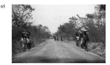
The pedestrians on this unpaved road have no option but to walk on the riding surface, close to moving traffic. Unless the grass is cut, the verge widened or a separate footpath formed, they are unable to avoid conflict with traffic.
