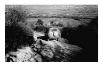
This steep hill on clay soil is difficult to ascend when dry and impossible when wet. The hill is suitable for spot improvement with an improved surface.
