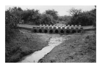
This photograph shows a causeway or vented drift. The raised blocks act as depth and width guides when in flood. They are spaced so that they can act as stepping stones for pedestrians. The inside edges are chamfered so as not to damage vehicle tyres or trap water-borne debris.
