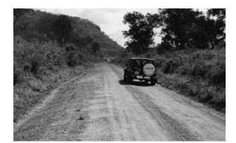
Grass is establishing itself naturally on this shoulder. Grass can be deliberately planted (see the earlier photograph of a scour check) or topsoil can be added to encourage natural grass. One danger of maintaining road surfaces with a grader is that this protective grass may be removed.
