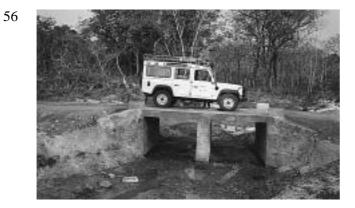
This small bridge has a mass concrete base slab, masonry abutments and pier and a reinforced concrete deck. The deck was cast using local timber formwork and falsework. Decks can also be made of dressed timber. Timber is easy to obtain in many areas, uses local suppliers and is easier to construct than a concrete deck. If the timber deck is built without load spreaders or running strips, it is easy to inspect for damage or rot.
