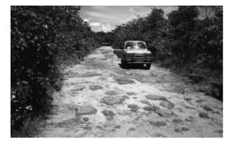
Surface material has worn away from this track to reveal rounded lateritic bedrock. The track is stable and passable at low speed. Removing the rock or forming a stable camber over the rock with imported material will be difficult and expensive. Unless the bedrock extends over a long length, severely disrupts traffic or damages tyres, leaving the track in its current condition may be the best solution.
