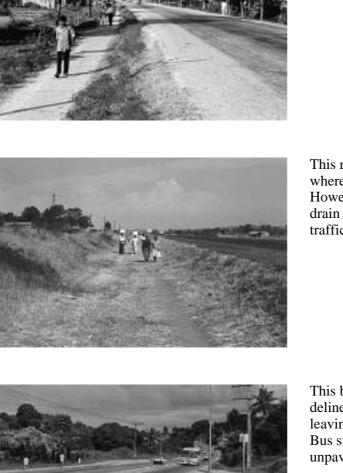
This footpath has been built several metres from moving traffic. The distance, the drain and the added height protect pedestrians from vehicles although it is noted that the deep and steep sided drain may trap vehicle wheels. This is a relatively high cost solution.
