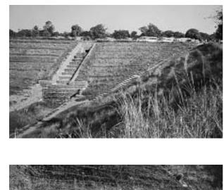
This deep erosion gully was formed during a few days of intense rain. After some rehabilitation landscaping, the slopes were protected against further erosion with contoured vegetation. In the right hand corner, a set of concrete steps should prevent pedestrians wearing out a channel which may initiate erosion, while the main structure is a gabion cascade bringing the water course down to a gabion protected channel in the base.
