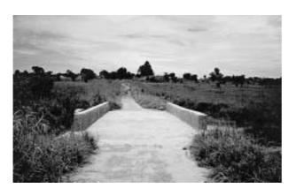
This small bridge on a track provides reliable and safe access across a stream. Since the track either side of the crossing is passable year round, the bridge is a worthwhile spot improvement.
