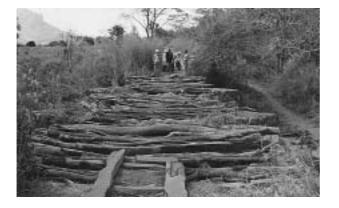
This rough log deck has been built on the abutments and piers of an earlier structure. It is in danger of imminent collapse and every crossing places the vehicle and passengers at great risk. A poorly built deck such as this can also restrict the water flow, leading to overtopping, and should be replaced as a matter of urgency.
