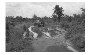
The soil along this rutted track is fine and poorly draining, so water ponds in any depression and the soil is pulverised into mud. The track becomes impassable, and every vehicle passage makes the condition worse. In dry weather, the resulting ruts are deep and hard to pass. The track should be locally raised and well cambered to prevent water ponding on the riding surface.
