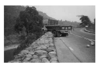
This truck was prevented from a very long fall by a barrier of gabions. Filled with stones and tied together with wire, gabions can form a very effective edge barrier.
