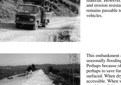
Despite traffic, flowing water and a total loss of camber, this steeply inclined stone surface remains stable and accessible. Improved surfaces are suitable for use as spot improvements on steep sections which would otherwise rapidly become impassable.
