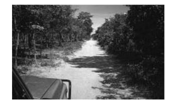
This track has no drains or camber. However, because of the low traffic levels, the well draining soil, the gentle slopes, the non-flooding terrain and vegetation which strengthens the soil, it is stable and strong and requires minimal maintenance to keep open all year round.
