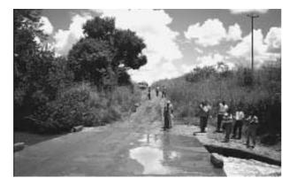
This ascent from a vented drift will often remain wet as water falls from passing vehicles. The gravel will therefore be weak and slippery. A short length of an improved surface will eliminate these problems and prevent access being lost.
