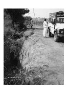
This side drain has become very severely eroded over many years without maintenance. The road is likely to collapse into the void and road users are in great danger. The erosion damage must be repaired, and scour checks and mitre drains installed.
