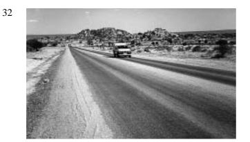
This road has been surfaced with an Otta seal. Bitumen is sprayed onto the base, a graded aggregate is spread onto the bitumen and the surface is then rolled with pneumatic tyred rollers to move the bitumen up through the aggregate. The sand along the side of the road is the residue from a blinding operation which is often required in the months after construction if excess bitumen moves up under the effect of traffic.
