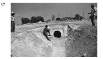
This photograph shows a well protected culvert outfall. There is no route for water to cut around the wingwalls. The outfall channel is built to a gradient of around 2% which should prevent erosion further downstream.
