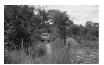
This is an overgrown but stable track. The woody stumps found between the wheeltracks should be removed to prevent damage to bicycle and car tyres. The high vegetation should also be cut to improve visibility and to reassure pedestrians afraid that snakes may be hiding in the grass.
