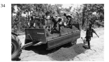
A typical construction site where labour based methods are used is likely to have tractors, trailers, twin drum pedestrian rollers and water bowsers. The sides of this trailer hinge down to make loading and unloading easier.
