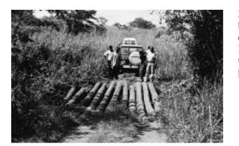
Logs can be used to construct an informal, but safe deck as in this photograph. This deck is not at risk of collapse, although the logs could have been placed closer together to make crossing easier for bicycles and pedestrians.
