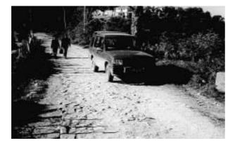
This photograph shows a stone surface. Large, dressed edge stones retain smaller, undressed stones and in doing so form a simple drain. The surface is also cambered to shed water. The surface is rough, but extremely durable. Repairs can be made very simply by removing the damaged area and relaying the stones.
