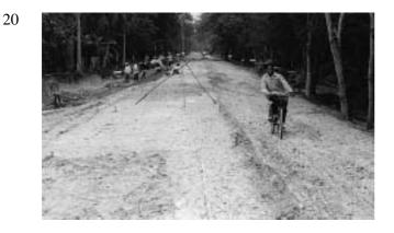
The fine soil on this road is dusty when dry and very slippery when wet. Gravel is hard to find in this area, so an improved surface, bituminous or non-bituminous, is recommended.
