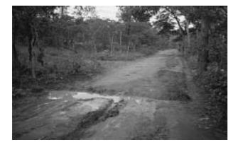
This diversion bank traps water running down the track and diverts it off the carriageway into side drains. Being drier, the track downhill remains in reasonable condition. Diversion banks are a very low cost improvement measure. They also serve to reduce traffic speed. They can be made of compacted soil, stones or logs. The bank in the photograph should have been constructed diagonally across the track so that water is not trapped in ruts in the wheel tracks.
