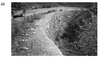
In hilly terrain, a substantial structure may be required to both support a culvert pipe and span a short gully. This structure has been built using locally available materials.
