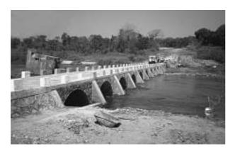
Simple techniques can be used to construct long bridges. This bridge uses masonry and reinforced concrete to cross a wide seasonal river. It is submersible and has flared piers with no parapet railings to help debris pass over the top. The earlier structure can be seen in the background – its higher level was perhaps unable to shed debris and contributed to its failure. The new structure was built using labour based methods by a contractor within a formal training programme.
