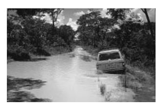
This track passes through an area which floods in the rainy season. Large ponds may be present year round, and during the rains the entire route is under water. Year round access can only be provided by a very expensive and long embankment. The road is nearly 100 km long, which may justify providing a Full standard (see Table 3.10).
