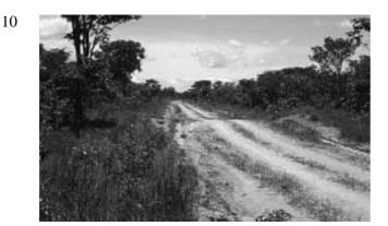
This road was formed from a stable track. However, the soil is light and non-plastic and the little vegetation which has grown is unable to give strength to the road structure. With no maintenance, it is likely that the road will return to a track in a short time. If access had been a priority, the track may have been left as it was. This illustrates how forming a track into a road can impose a maintenance burden on an under-resourced Road Manager.
