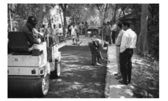
This photograph shows a thin seal being constructed using labour based methods on a broken brick water bound macadam base. Aggregate and bitumen are heated and then mixed over fire. The mix is transported by bicycle, spread manually to the thickness of thin spacer bars and compacted by a vibrating twin drum roller.
