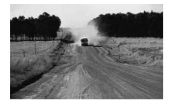
This photograph shows the level of dust that can be generated from a gravel road. The dust brings health problems to villages, affects agricultural output, is dangerous when vehicles pass or attempt to overtake and demonstrates why gravel must be frequently replenished. (Photograph courtesy of CSIR, South Africa)
