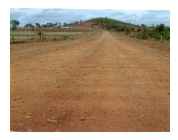
Patching is not a satisfactory method of repairing **corrugations. Grading** (Part A) or labour based reshaping (Part B) should be used to repair these defects.
