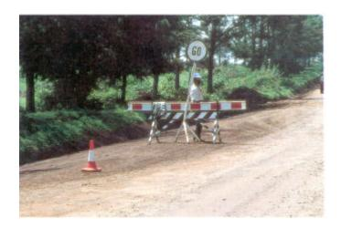
m **Traffic controllers** should stand next to the barriers in the centre of the road to operate the reversible "Stop/Go" signs.
