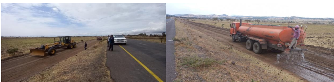
Figure 16 Construction of temporary diversion road to facilitate construction of MECS and chipseal control sections.
