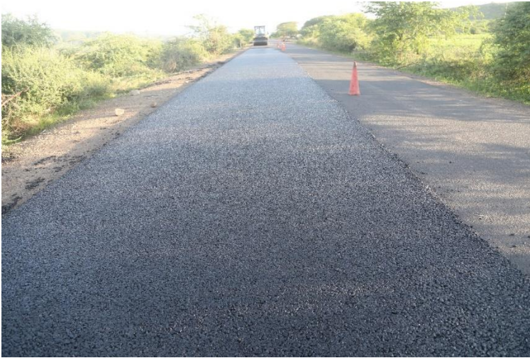
Figure 24 Completed FMA trial section.
