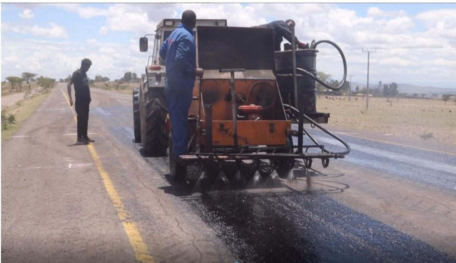
Figure 19 Epoxy binder application for MECS
