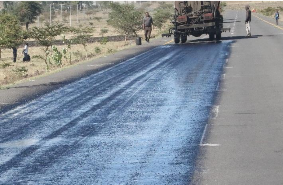
Figure 20 Bitumen binder application for the control section
