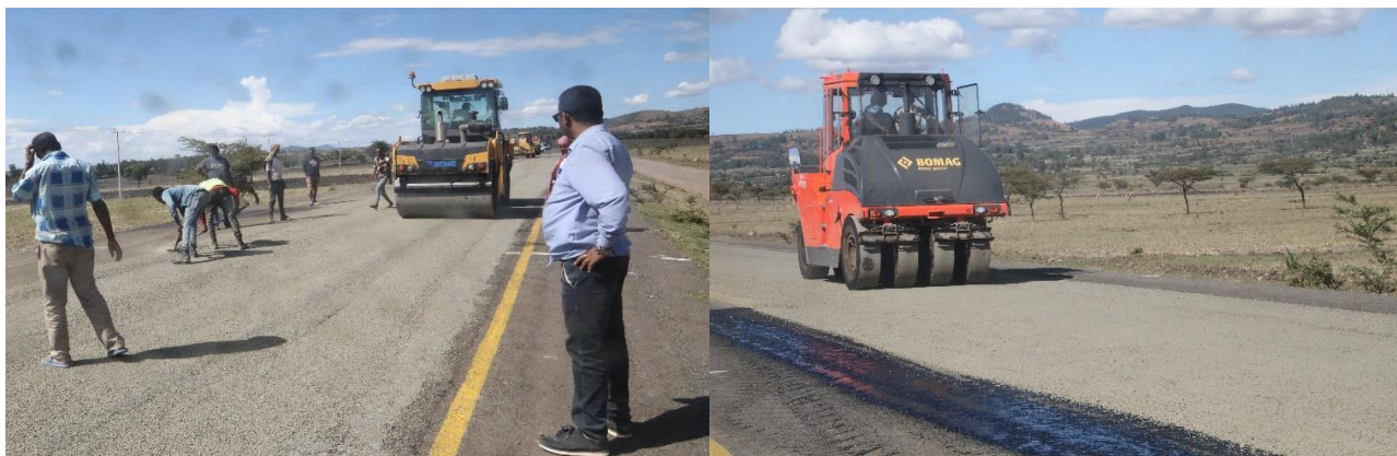
Figure 22 Compaction of the chipseal surface
