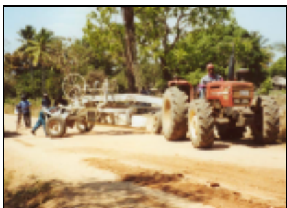
Plate 10 Tractor towed scarification
