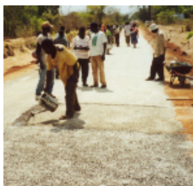
Plate 13 Application of binder using watering can
