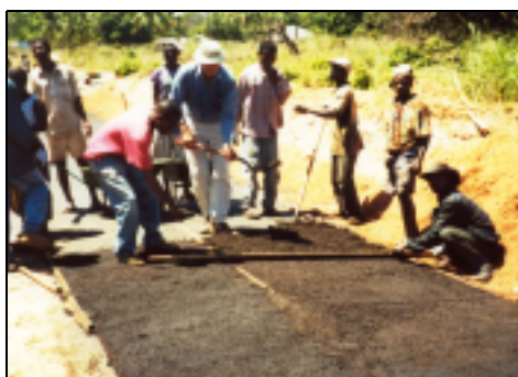
Plate 16 Placing of material between wooden batons.
