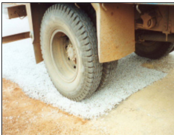
Plate 6 Lorry wheel compaction
