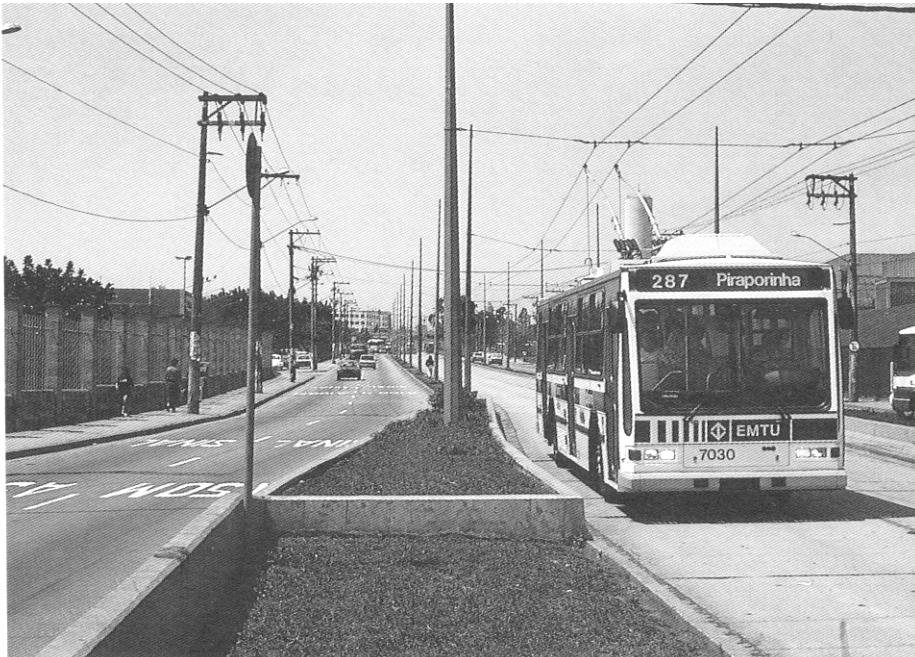
Plate 7 Median busway using the central reserve of a dual carriageway: Sao Paulo
