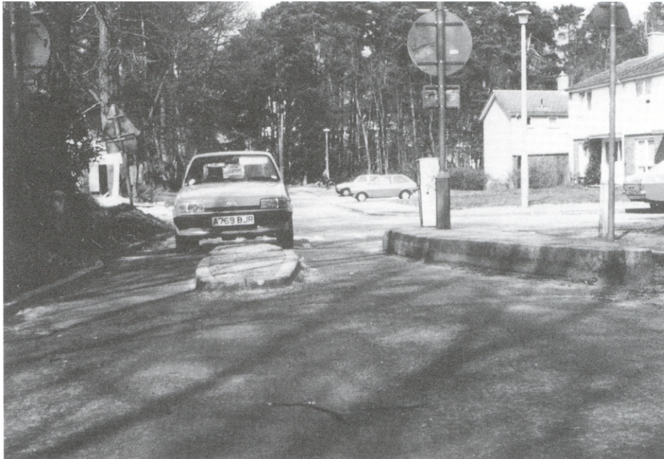
Plate 15 Busway entry barrier
