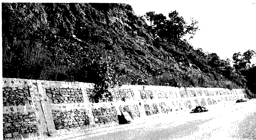
Plate 5 Mortared-framed masonry wall, performing successfully
