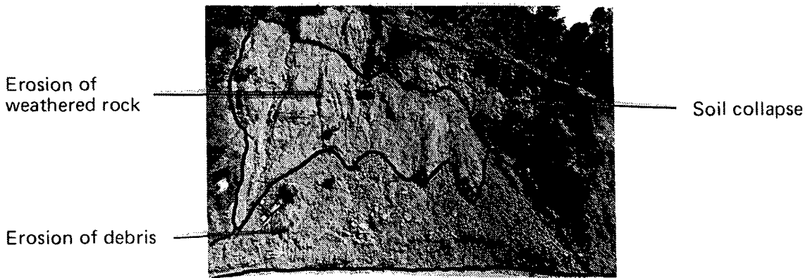
Plate 1 Modes of failure I
