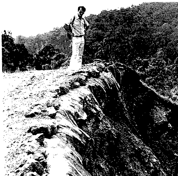
Plate 10 Roofing felt cover at head of landslide
