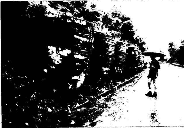
Fig 5 The first cylinder wall in the early stages of failure, four months into the first monsoon season. During the following few days progressive movement of the landslide led to the destruction of the wall along half its length
