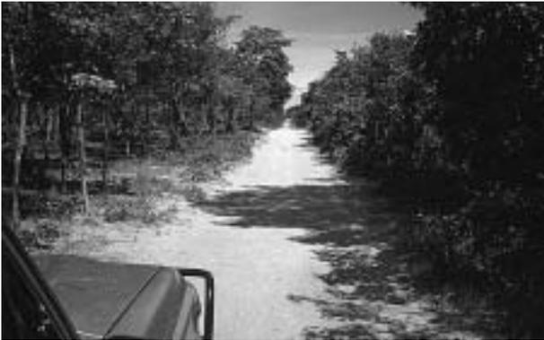
This track has no drains or camber. However, because of the low traffic levels, the well draining soil, the gentle slopes, the non-flooding terrain and vegetation which strengthens the soil, it is stable and strong and requires minimal maintenance to keep open all year round.
