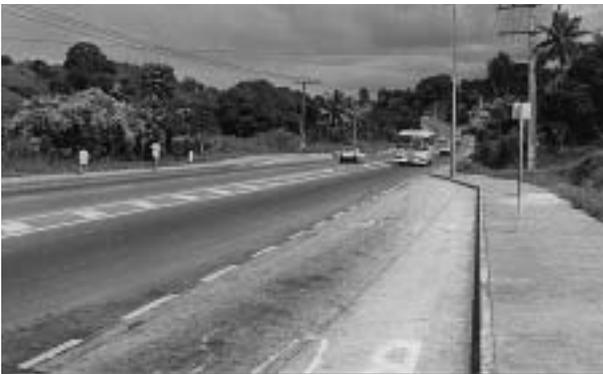
This bus stop lay-by is clearly marked and delineated from moving traffic. Those leaving the bus are protected from traffic. Bus stops such as this can be easily made on unpaved rural roads.
