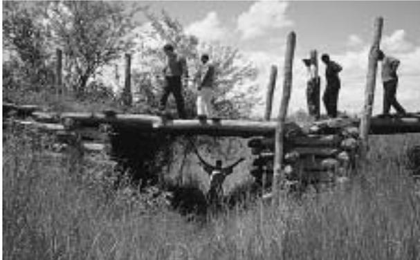
This bridge is constructed entirely from stripped logs. It survived floods which destroyed a number of nearby pipe culverts and remained fully passable.
