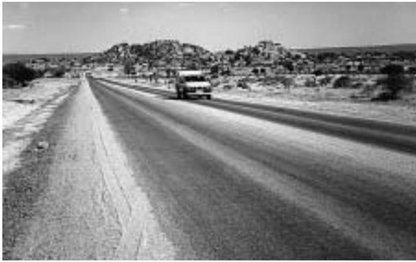
This road has been surfaced with an Otta seal. Bitumen is sprayed onto the base, a graded aggregate is spread onto the bitumen and the surface is then rolled with pneumatic tyred rollers to move the bitumen up through the aggregate. The sand along the side of the road is the residue from a blinding operation which is often required in the months after construction if excess bitumen moves up under the effect of traffic.
