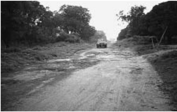
A side drain on this secondary road has become blocked with sediment. Water has overtopped, cut across the carriageway and caused significant damage. Deterioration will continue until the drain is cleared and water properly disposed of. Similar problems can occur if road users block drains in order to access road side properties. If this happens, the Road Manager should explain to road users the problems caused by blocking drains and then help them form small culverts to access their properties.
