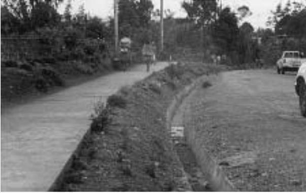
This footpath has been built several metres from moving traffic. The distance, the drain and the added height protect pedestrians from vehicles although it is noted that the deep and steep sided drain may trap vehicle wheels. This is a relatively high cost solution.
