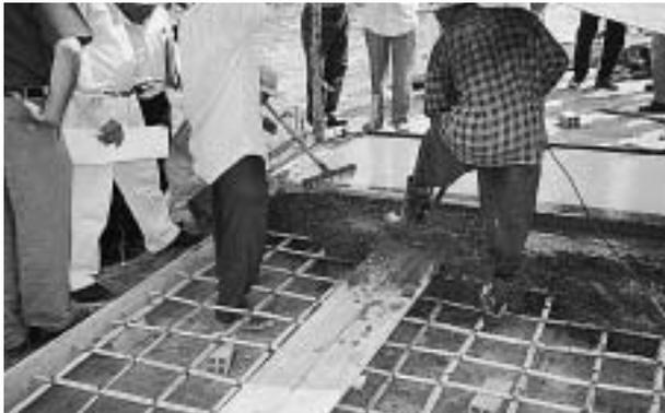
A concrete surface is very strong, but steel reinforcing bars make it very expensive. Bamboo strips are proving to be a suitable low cost alternative to steel bars.
