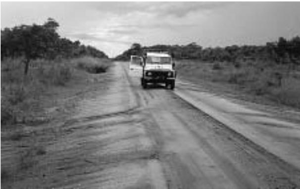
This road has been well formed. However, inadequate maintenance has left ruts in the wheel tracks while the poor quality gravel has little resistance to erosion. The ruts concentrate water and form gullies in the shoulders. More frequent grading or rut filling of the surface and vegetation on the shoulders would reduce the gullying. Unless resolved, the problem will worsen and access will eventually be lost.
