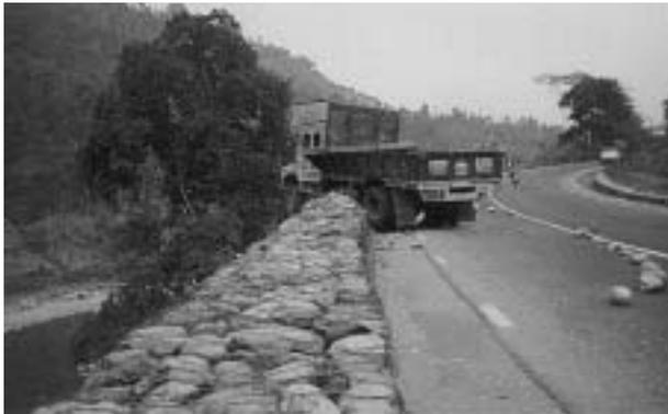
This truck was prevented from a very long fall by a barrier of gabions. Filled with stones and tied together with wire, gabions can form a very effective edge barrier.
