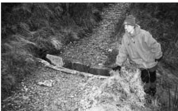
This narrow stone lined channel allows pedestrians to cross a stream with ease and prevents erosion of the footpath. It is a very low cost improvement. If the hillside below the path were prone to erosion, an outfall structure would be required. The channel can also collect and dispose of water that might flow down the footpath itself.
