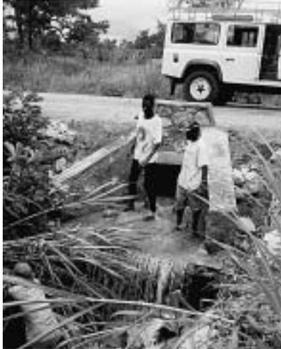
Erosion began in this culvert outfall channel some distance downstream. The erosion has moved upstream and is now undercutting the apron, putting the entire structure at risk of collapse. Run-off around the wingwalls has contributed to the problem. The downstream erosion needs to be controlled by reforming the channel and constructing scour checks. Then any structural damage should be repaired, and the wingwalls extended down to apron level and backfilled.
