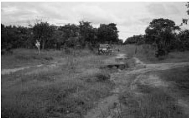
Run off from the surrounding land is causing serious erosion to this very badly maintained road. It is necessary to protect the inside face of the side drain or to dig interception drains to channel the water to a water course or a culvert. Interception ditches are more effective than drain lining, but maintenance can often be overlooked if they are out of sight.
