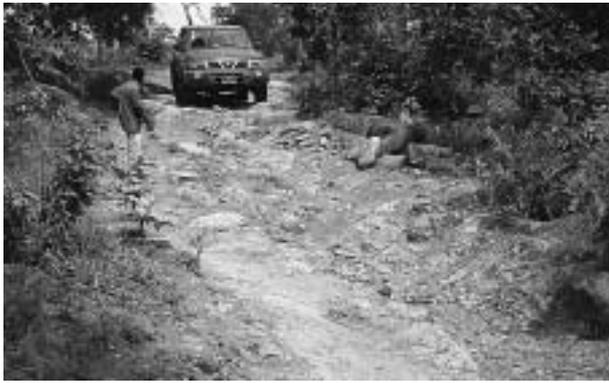
Four wheel drive passage down this extremely rocky track is very slow and requires great care, while the vehicle, particularly the tyres, can be damaged. This track is clearly not providing safe and reliable access. Providing access will require major improvement work or route realignment.
