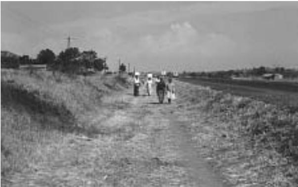
This road has been built with wide shoulders where pedestrians can walk safely. However, in the dry season, the wide side drain provides even greater safety from traffic.
