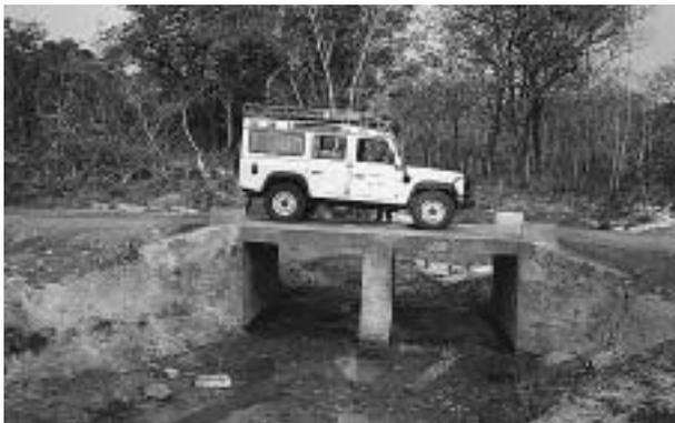
This small bridge has a mass concrete base slab, masonry abutments and pier and a reinforced concrete deck. The deck was cast using local timber formwork and falsework. Decks can also be made of dressed timber. Timber is easy to obtain in many areas, uses local suppliers and is easier to construct than a concrete deck. If the timber deck is built without load spreaders or running strips, it is easy to inspect for damage or rot.
