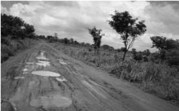
A camber is required to shed water from a carriageway. This secondary road has not been graded for a long time, the camber has been lost and potholes are developing. Each vehicle passage worsens the situation. The road should be reshaped as soon as possible.
