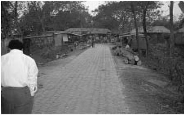
This embanked road has been surfaced with two layers of bricks in a herringbone pattern. The manufacture of these bricks uses local clay and local skills, although there are concerns of excessive wood use in the kilns. When an upgrade is planned, the bricks can be lifted, manually broken and used as a water bound macadam base below a bituminous seal.
