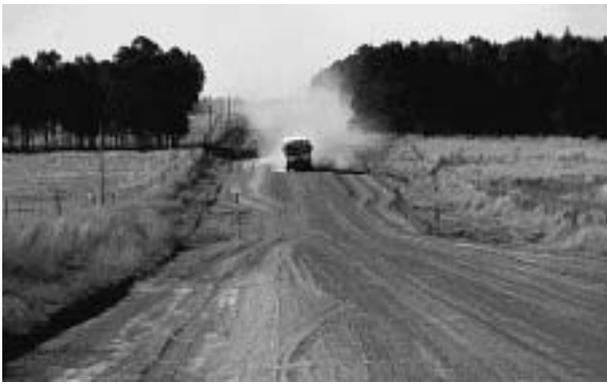
This photograph shows the level of dust that can be generated from a gravel road. The dust brings health problems to villages, affects agricultural output, is dangerous when vehicles pass or attempt to overtake and demonstrates why gravel must be frequently replenished. (Photograph courtesy of CSIR, South Africa)
