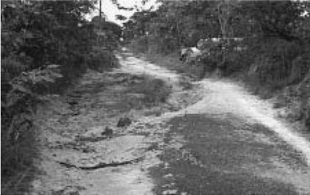
Rain falling on the surface of this inclined track flows down the gradient forming small erosion channels. Little water absorbs into the well compacted fine soil. The channels concentrate the water and can grow into severe longitudinal erosion. The track has become impassable and vehicles must detour through the undergrowth. The track should be reformed with camber, side drains and mitre drains or the solution shown below can be used.
