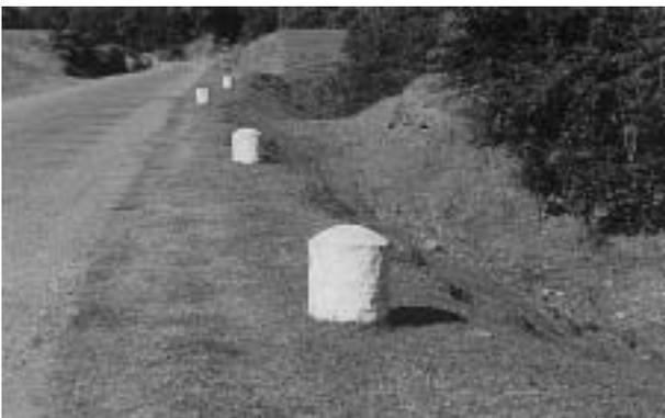
This photograph shows low cost edge delineators being used to indicate a steep drop. They are made from half-buried oil drums filled with sand and capped with concrete. They are painted white for greater visibility, particularly at night.
