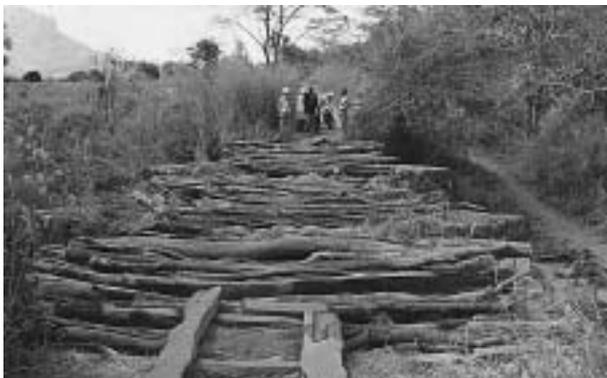
This rough log deck has been built on the abutments and piers of an earlier structure. It is in danger of imminent collapse and every crossing places the vehicle and passengers at great risk. A poorly built deck such as this can also restrict the water flow, leading to overtopping, and should be replaced as a matter of urgency.
