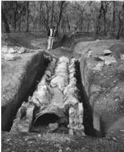
Culverts can be built in many ways. Pipes of corrugated galvanised sheet can be installed quickly but are expensive and often hard to obtain. This culvert is built with a wet masonry arch over removeable pipe formwork, thereby reducing the reliance on imported materials. It was necessary to convince the masons, using wooden shaped blocks, that the arch would stand when the formwork was removed, but once convinced, they quickly adopted their new skills.
