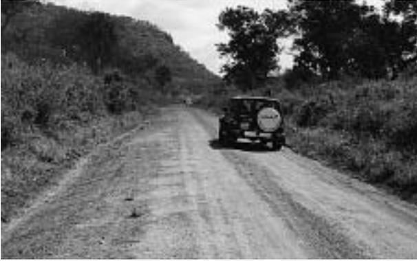
Grass is establishing itself naturally on this shoulder. Grass can be deliberately planted (see the earlier photograph of a scour check) or topsoil can be added to encourage natural grass. One danger of maintaining road surfaces with a grader is that this protective grass may be removed.
