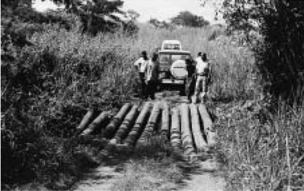
Logs can be used to construct an informal, but safe deck as in this photograph. This deck is not at risk of collapse, although the logs could have been placed closer together to make crossing easier for bicycles and pedestrians.
