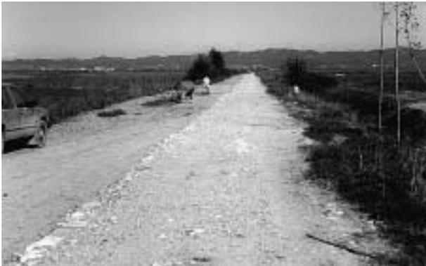
This embankment across low lying and seasonally flooding land has a stone surface. Perhaps because of disruption to the works, perhaps to save funds, only half has been surfaced. When dry, the full width is accessible. When wet, the surfaced half provides reliable access.
