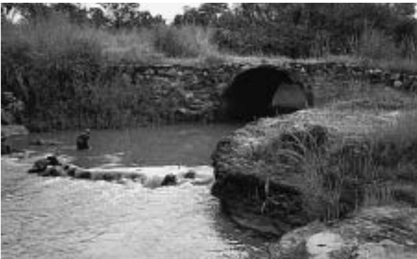
This culvert has minimal cover over a large diameter corrugated sheet pipe. The surface of the pipe is visible from above. Lack of cover is a problem for a normal small diameter culvert, but here it could cause sudden collapse and loss of life. The culvert should be inspected carefully and adequate cover provided as a matter of urgency.
