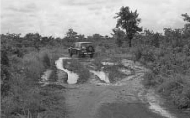
The soil along this rutted track is fine and poorly draining, so water ponds in any depression and the soil is pulverised into mud. The track becomes impassable, and every vehicle passage makes the condition worse. In dry weather, the resulting ruts are deep and hard to pass. The track should be locally raised and well cambered to prevent water ponding on the riding surface.
