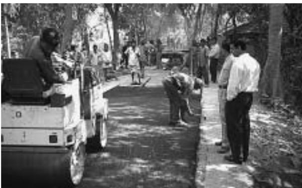
This photograph shows a thin seal being constructed using labour based methods on a broken brick water bound macadam base. Aggregate and bitumen are heated and then mixed over fire. The mix is transported by bicycle, spread manually to the thickness of thin spacer bars and compacted by a vibrating twin drum roller.
