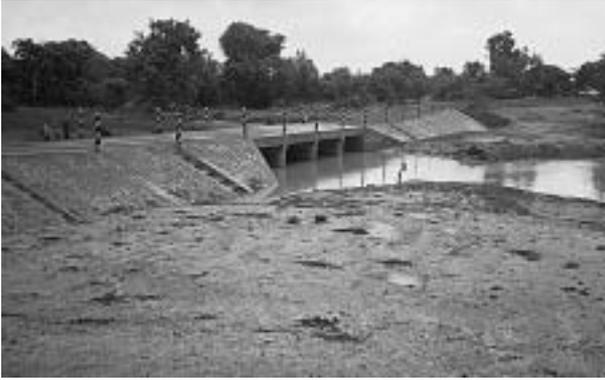
In many situations, a road may cross a water course and then continue across low lying land. An isolated bridge would cross the water course, but embankments are needed to provide access along the entire route. This photograph shows a submersible bridge between embankments that will provide year round access.
