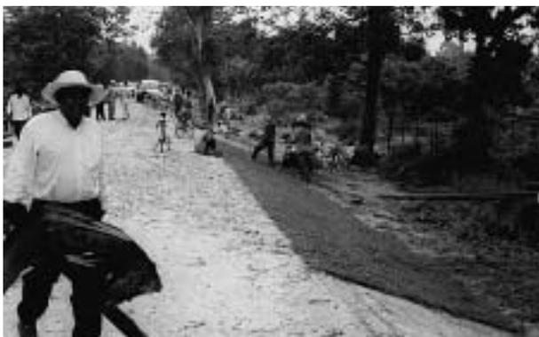
Slopes often erode if they are steep and unprotected. Turf is being laid on this embankment to protect it from erosion. The turf was grown in a nursery specifically for this use.
