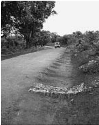
This photograph, looking downhill, shows a scour check to reduce erosion. It is well built with wooden stakes and stones and well shaped to keep the water flowing in the centre of the drain. A mitre drain was dug at the bend in the road but more should have been dug to divert the water onto the surrounding land. Grass has also been planted along the shoulder line in an attempt to prevent erosion.
