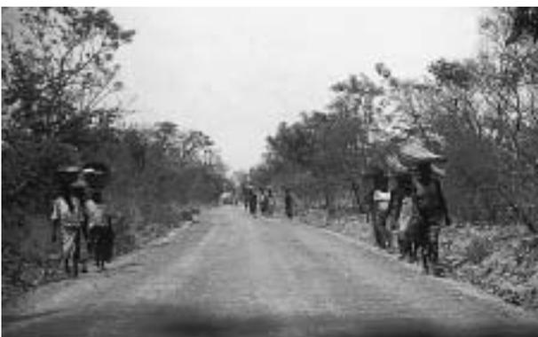
The pedestrians on this unpaved road have no option but to walk on the riding surface, close to moving traffic. Unless the grass is cut, the verge widened or a separate footpath formed, they are unable to avoid conflict with traffic.
