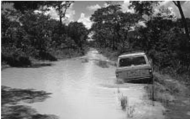
This track passes through an area which floods in the rainy season. Large ponds may be present year round, and during the rains the entire route is under water. Year round access can only be provided by a very expensive and long embankment. The road is nearly 100 km long, which may justify providing a Full standard (see Table 3.10).
