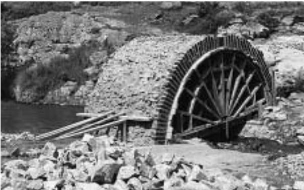
A masonry arch can be constructed to a larger size than in the above photograph, as in this structure with a span of around 5 metres. The formwork must be very carefully constructed.
