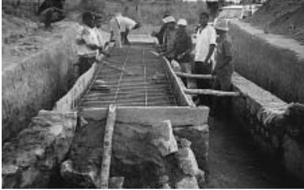
This double culvert has masonry walls upon which a reinforced concrete cover slab is being built. Previously excavated soil is used as formwork for the cover slab and will be removed when the concrete has gained sufficient strength.
