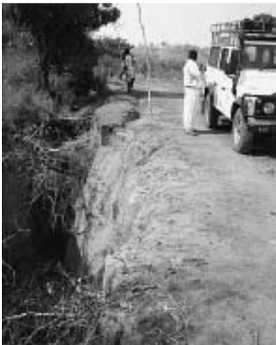
This side drain has become very severely eroded over many years without maintenance. The road is likely to collapse into the void and road users are in great danger. The erosion damage must be repaired, and scour checks and mitre drains installed.
