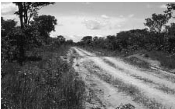
This road was formed from a stable track. However, the soil is light and non-plastic and the little vegetation which has grown is unable to give strength to the road structure. With no maintenance, it is likely that the road will return to a track in a short time. If access had been a priority, the track may have been left as it was. This illustrates how forming a track into a road can impose a maintenance burden on an under-resourced Road Manager.
