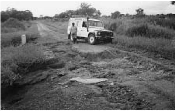
It is important to correctly determine the flow requirement of a culvert. This single aperture culvert was built without consideration of the catchment area and potential run off volume. In a single storm it overtopped and rendered the road accessible to only four wheel drive vehicles.
