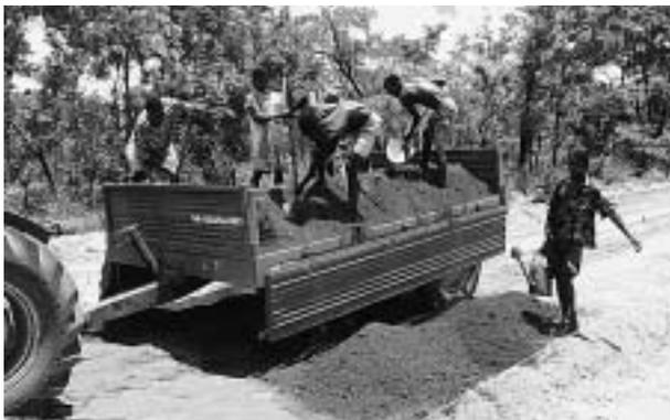
A typical construction site where labour based methods are used is likely to have tractors, trailers, twin drum pedestrian rollers and water bowsers. The sides of this trailer hinge down to make loading and unloading easier.
