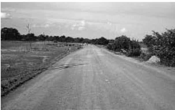
This secondary road is well maintained, but is very wide. The carriageway will collect a large amount of rainfall and it will be difficult to maintain a camber. Despite the obvious recent maintenance, the crown is flat and small potholes are already developing. Roads are often prepared in this way ready for a seal, but the seal is often not completed.
