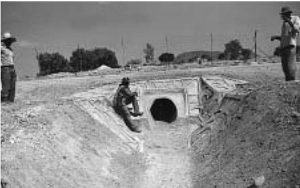
This photograph shows a well protected culvert outfall. There is no route for water to cut around the wingwalls. The outfall channel is built to a gradient of around 2% which should prevent erosion further downstream.
