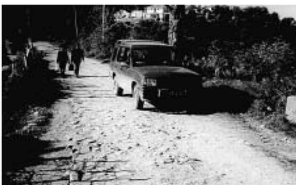
This photograph shows a stone surface. Large, dressed edge stones retain smaller, undressed stones and in doing so form a simple drain. The surface is also cambered to shed water. The surface is rough, but extremely durable. Repairs can be made very simply by removing the damaged area and relaying the stones.
