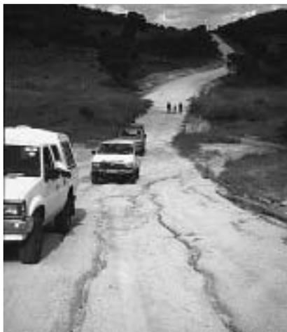
Longitudinal erosion is beginning to form deep gullies in this carriageway. Maintaining the camber with regular grading would have prevented this happening, although that is hard to do on a carriageway as wide as this.
