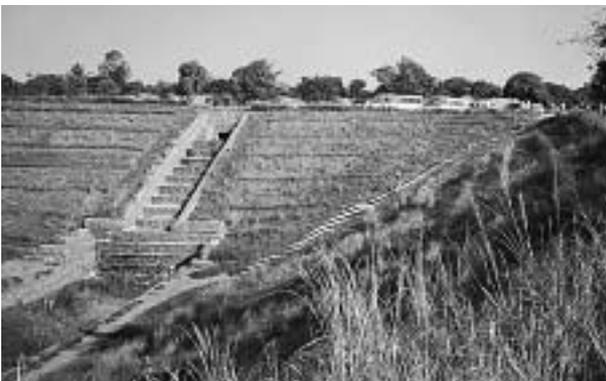
This deep erosion gully was formed during a few days of intense rain. After some rehabilitation landscaping, the slopes were protected against further erosion with contoured vegetation. In the right hand corner, a set of concrete steps should prevent pedestrians wearing out a channel which may initiate erosion, while the main structure is a gabion cascade bringing the water course down to a gabion protected channel in the base.
