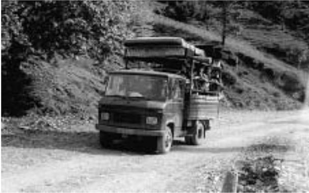
A stone surface remains passable for many years. This surface has lost all shape as the stones have been pressed into the base material. However, the stones give strength and erosion resistance to the base, which remains passable to a wide variety of vehicles.
