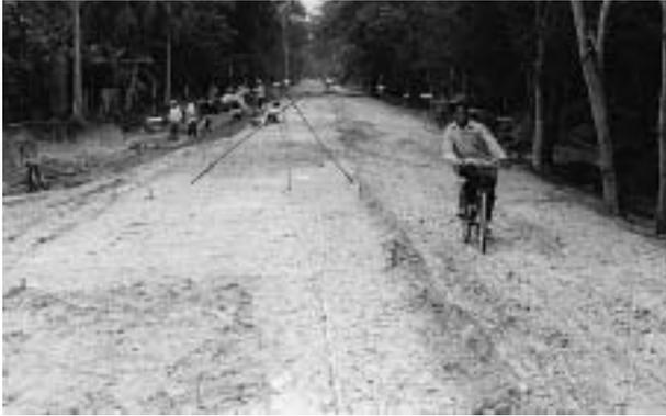
The fine soil on this road is dusty when dry and very slippery when wet. Gravel is hard to find in this area, so an improved surface, bituminous or non-bituminous, is recommended.
