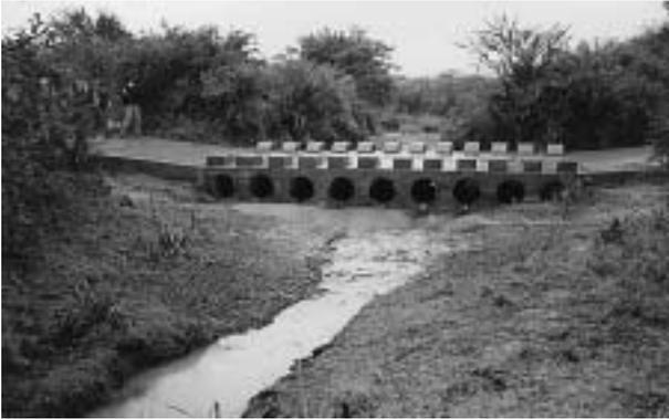
This photograph shows a causeway or vented drift. The raised blocks act as depth and width guides when in flood. They are spaced so that they can act as stepping stones for pedestrians. The inside edges are chamfered so as not to damage vehicle tyres or trap water-borne debris.
