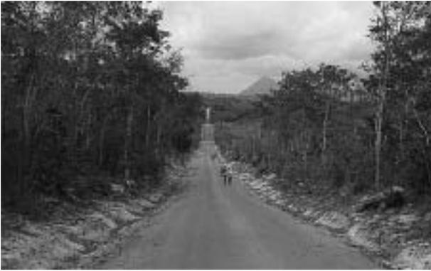
This photograph shows a good gravel road. It has a camber, side drains and mitre drains, although the latter are hard to see. With two or three years of vegetation growth on the shoulders and side slopes, the road will be more durable and erosion resistant.
