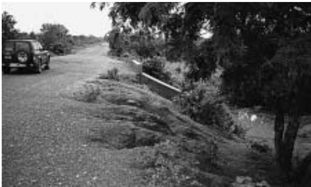
This road shoulder is badly eroded. The extent of erosion can be seen from the height of the wingwall, originally at ground level. Shoulder erosion often occurs near water crossings as water concentrates at the low point on the road surface and then runs off the shoulder. The shoulder should be reconstructed and vegetation planted on the steep slope.
