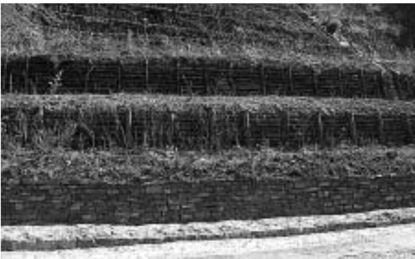
This combination of dry masonry retaining wall, timber crib walls and contoured planting has been constructed to stabilise a slope. After two years the measures were well rooted and secure. (Photograph courtesy of Ruth Schaffner, consultant, Oberhofen, Switzerland')
