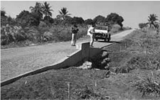
After the above culvert overtopped, it would have been disruptive and expensive to rebuild a higher capacity culvert. An easier solution was to repair the erosion damage and construct a downstream cut off wall as a weir. The culvert may overtop but the short length of road will act as a long drift. Gabions support the wall and have been topsoiled and grassed. The headwall was raised to reduce erosion close to the outfall.
