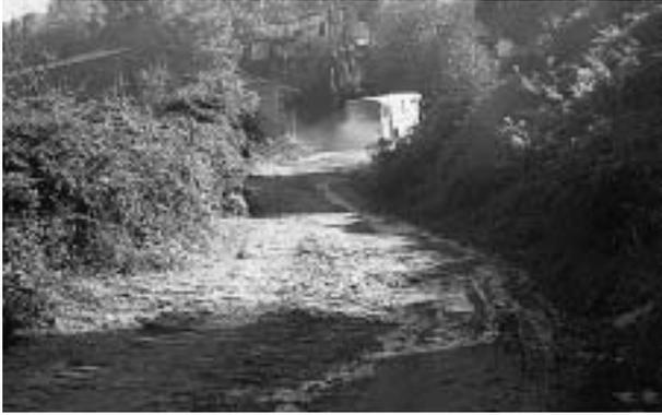
Despite traffic, flowing water and a total loss of camber, this steeply inclined stone surface remains stable and accessible. Improved surfaces are suitable for use as spot improvements on steep sections which would otherwise rapidly become impassable.
