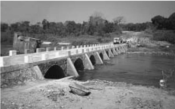
Simple techniques can be used to construct long bridges. This bridge uses masonry and reinforced concrete to cross a wide seasonal river. It is submersible and has flared piers with no parapet railings to help debris pass over the top. The earlier structure can be seen in the background – its higher level was perhaps unable to shed debris and contributed to its failure. The new structure was built using labour based methods by a contractor within a formal training programme.
