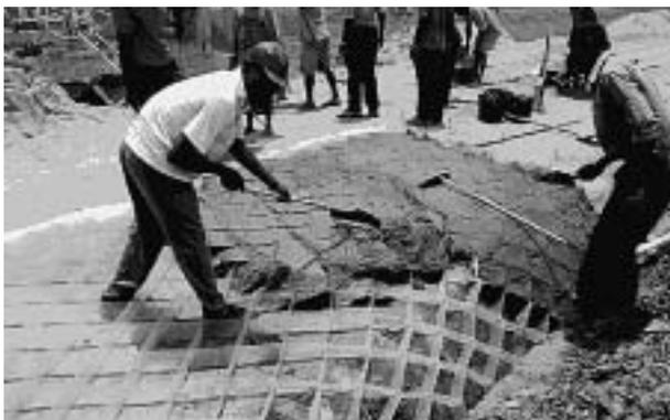
This photograph shows a proprietary system whereby a pre-formed grid of polythene strips is tensioned and filled with a cement stabilised sand. The result is a type of in-situ block pavement. The strips are profiled to form keys between blocks, allowing load to be transferred and the surface to flex without cracking. The polythene grid retains the blocks, removing the need for edge beams or kerbs. (Photograph courtesy of Scott Wilson Africa Limited)
