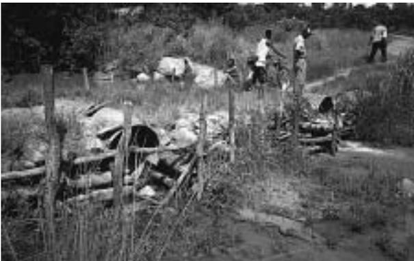
This multi-bore culvert takes a tertiary road across a water course. The culvert has not been well maintained and the few repairs carried out have been inadequate. The culvert is difficult and dangerous to cross and likely to be impassable in the rains. The culvert should be reconstructed to ensure access and safety.
