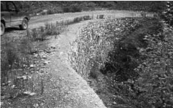
In hilly terrain, a substantial structure may be required to both support a culvert pipe and span a short gully. This structure has been built using locally available materials.
