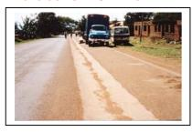
The parabolic dish drain has good hydro-dynamics but a low capacity. The capacity can be improved by deepening the parabola or by increasing the number of turn-outs. This style of drain is ideal for low rainfall situations or routes with a high number of roadside properties or accesses. A deeper drain can be constructed further away from the road to collect rainfall run-off from outlying land if required.
