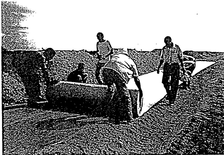
Geosynthetic material being laid as a drainage layer between sub-base and road base.
