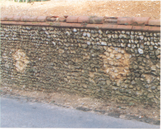
Figure 3: A photograph of a retaining wall constructed from dark, irregular stones, topped with a row of reddish-brown bricks. A paved road is visible at the bottom left.
