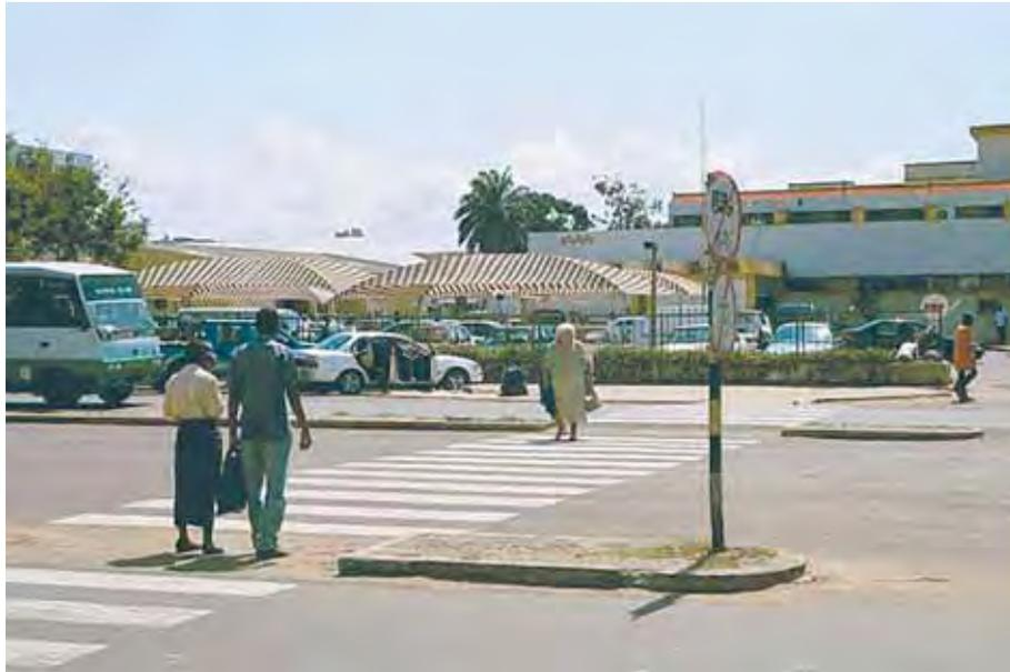
**Figure 3.20** Pedestrian crossing opposite hospital entrance with newly installed kerb ramps, cuts in central island and road marking installed as part of the demonstration project in Maputo, Mozambique (*Following the improvements, a huge increase in the proportion of elderly and ambulatory disabled people using the crossing was observed.*)
