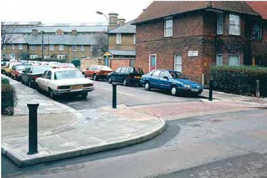
**Figure 3.21** Kerb extensions reduce the crossing width for pedestrians
