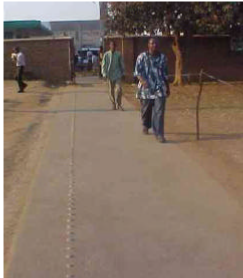
Figure 6: Upgraded footway with tactile path, Blantyre
