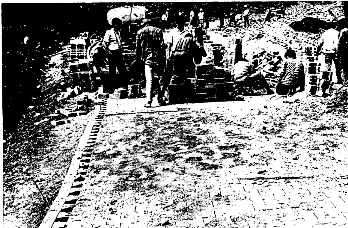
Plate 2 Concrete block pavement on steep gradient
