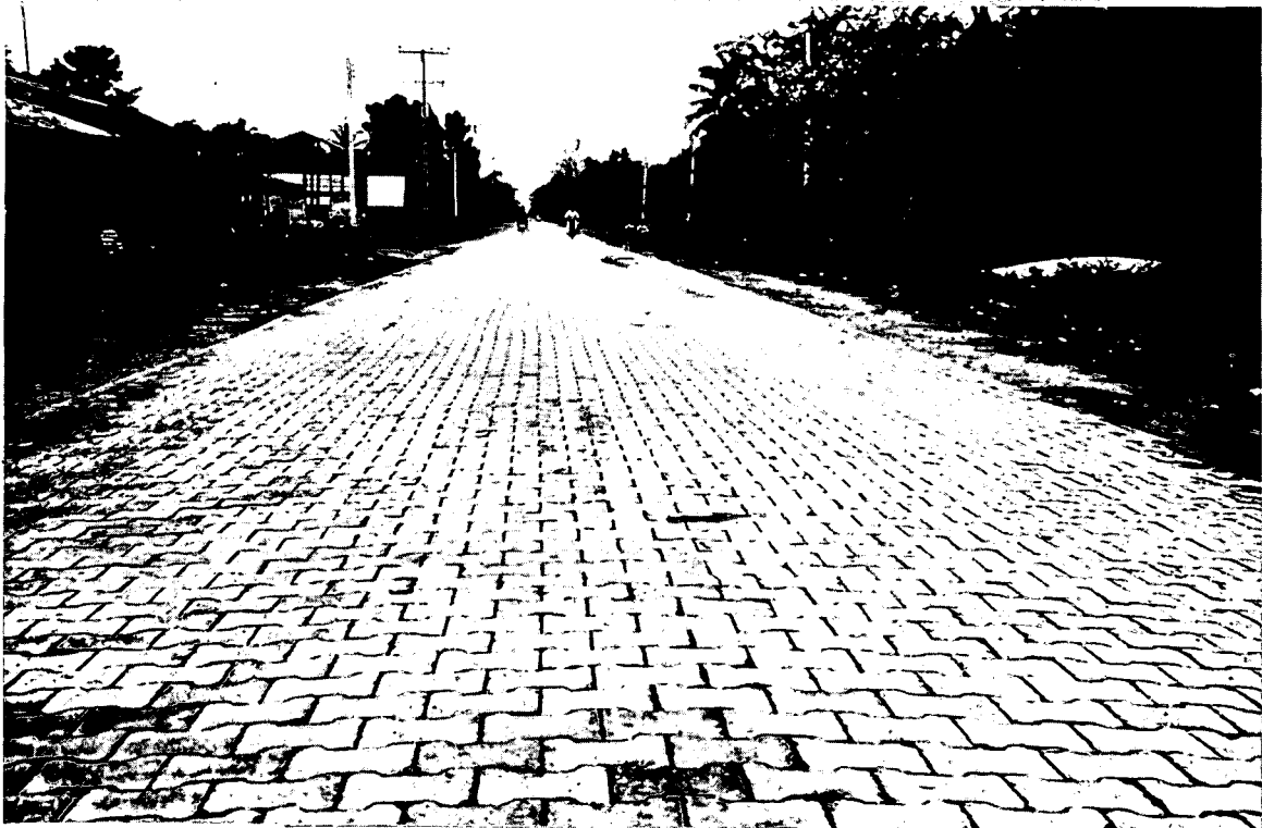
Plate 4 Concrete block pavement after 18 months trafficking
