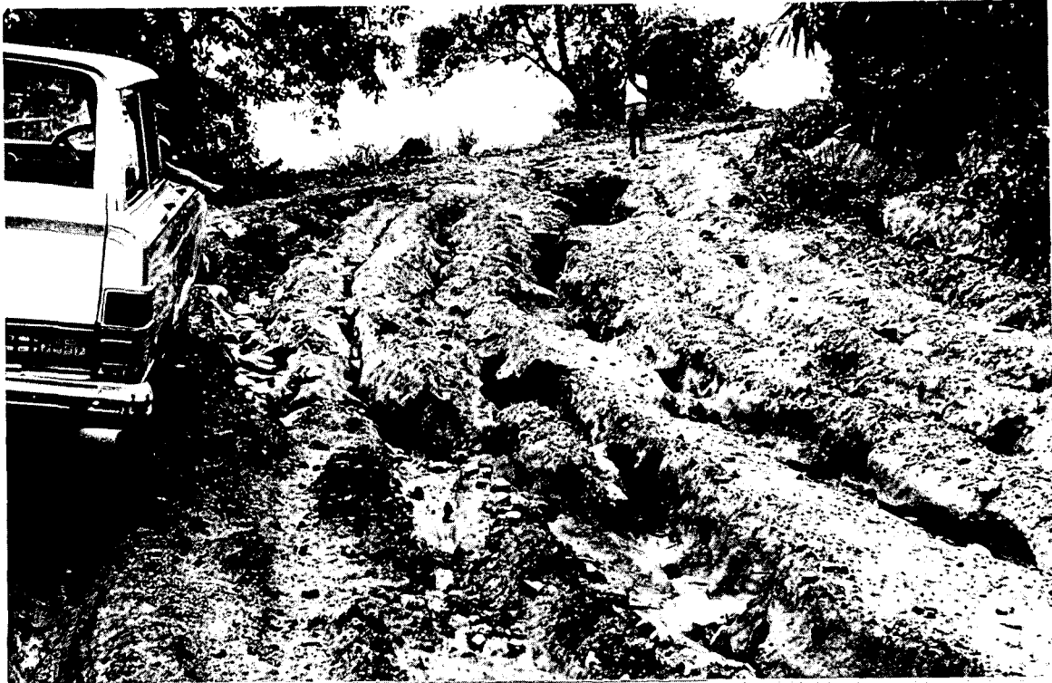
Plate 1 Erosion on steep gradient
