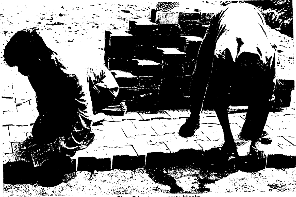
Plate 5 Laying concrete blocks
