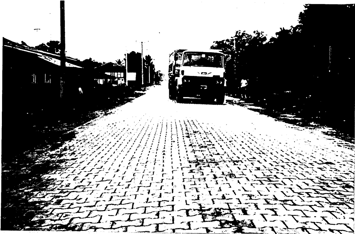
Plate 3 Heavy traffic on block pavement
