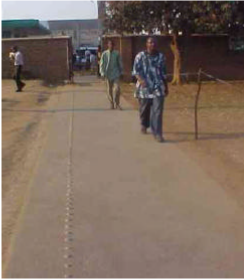
Figure 5: Upgraded footway with tactile path, Blantyre
