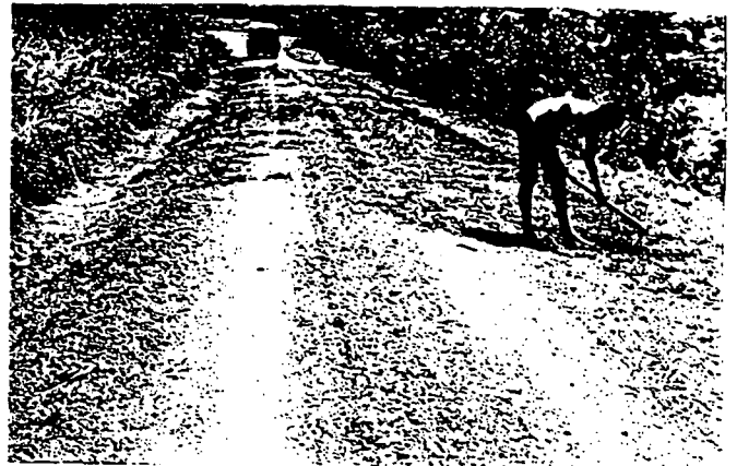
Plate 2. Grubbing edge
