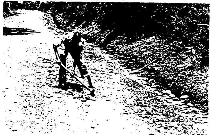
Plate 4. Re-shaping carriageway
