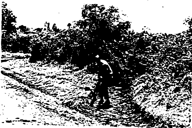
Plate 7. Cleaning mitre drain
