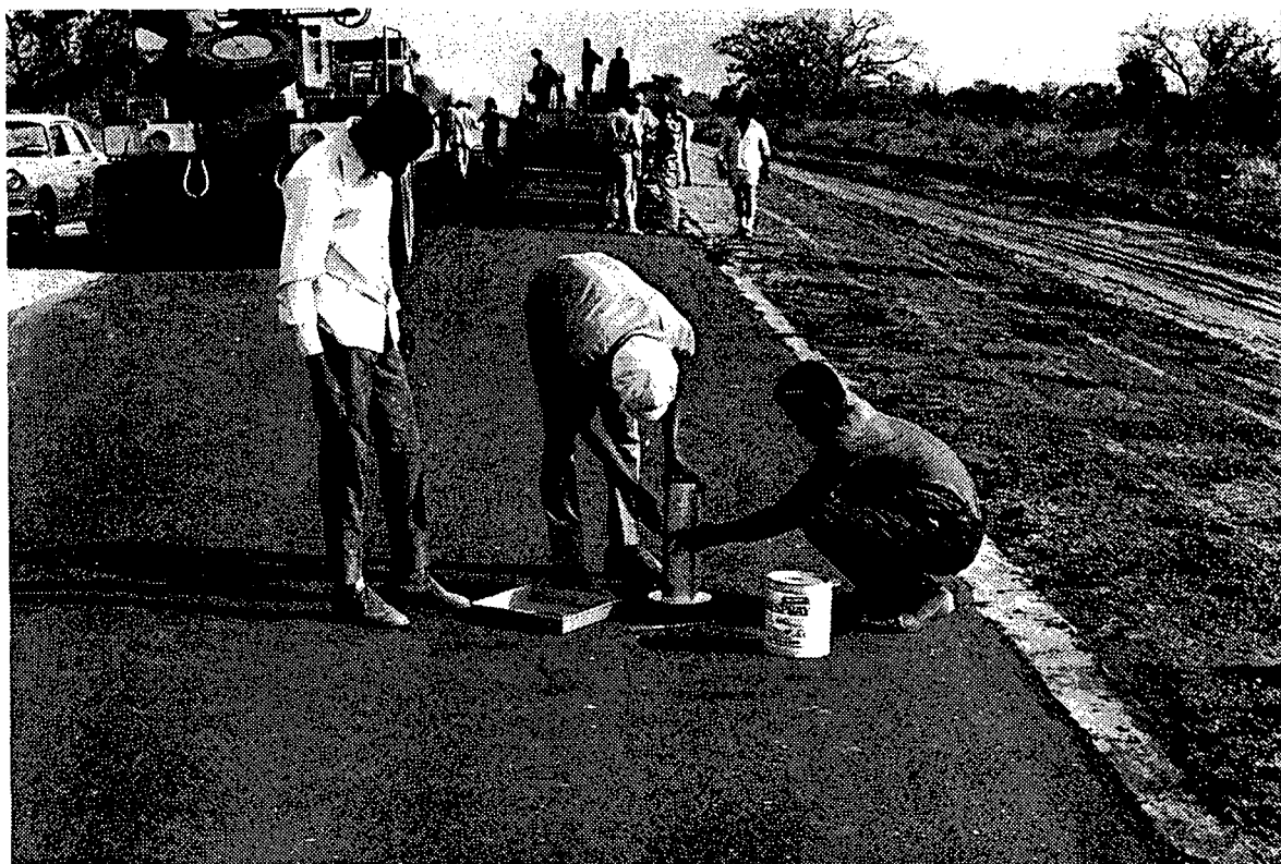
Fig. 10. Finished surface of sand-bitumen base
