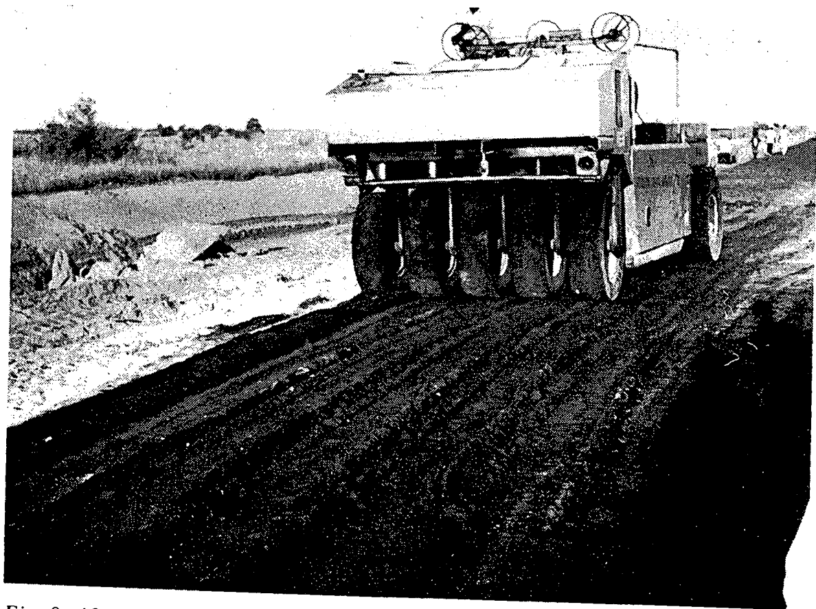
Fig. 9. 19 t pneumatic-tyred roller compacting sand-bitumen
