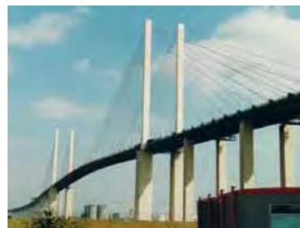
Figure 12.9: Cable stayed bridge
