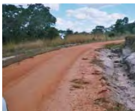
Figure 11.3: This side drain is eroding severely. Access along the road may soon be lost. Scour checks should be constructed
