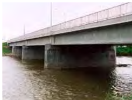
Figure 12.7: Pre-stressed beam and slab bridge
