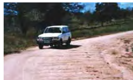
Figure 11.1: Transverse erosion on a super-elevated curve
