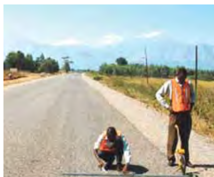
Figure 9.4: A good surface dressing
