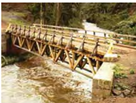
Figure 12.6: Modular timber bridge
