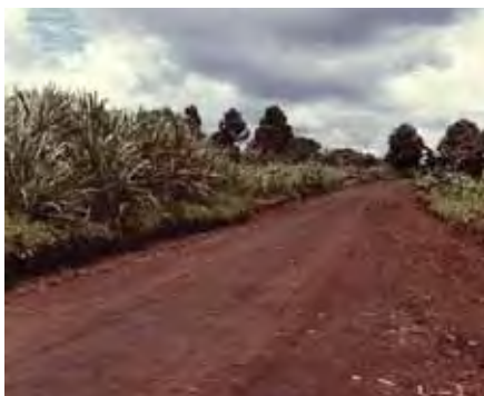
Figure 9.2: Well shaped earth road
