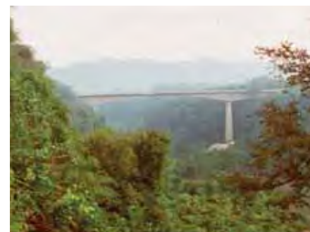
Figure 12.8: Concrete box girder bridge
