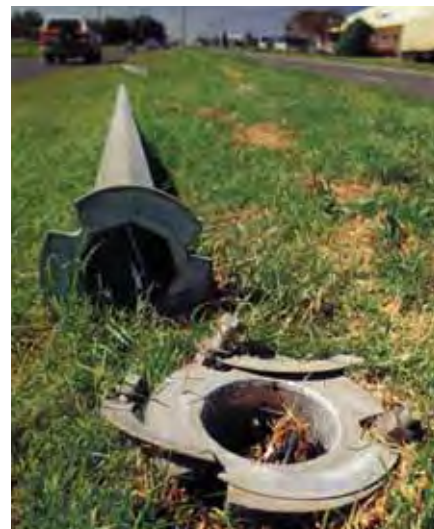
Figure 8.3: Frangible lamp post after vehicle collision, Australia
