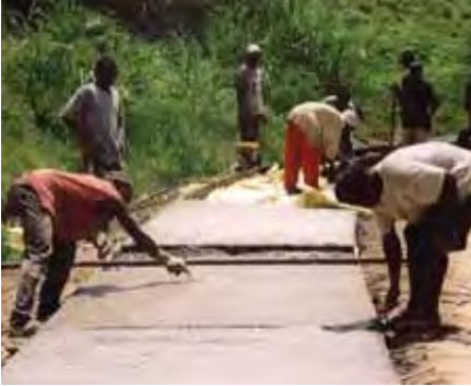
Figure 7.2: Labour-based road works, Tanzania
