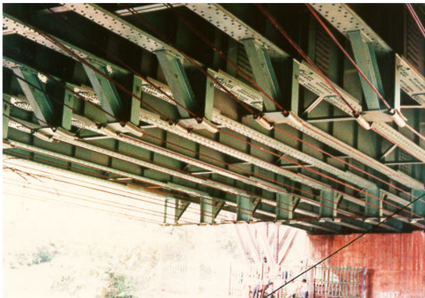
Figure 2 Condet Bridge after strengthening.
