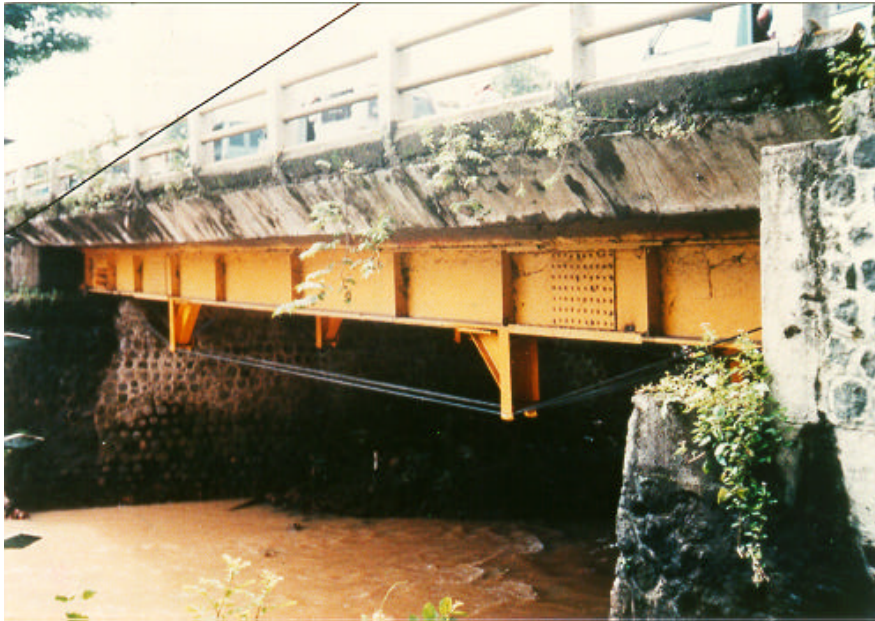
Figure 3 Kemlaka Gede bridge after strengthening.
