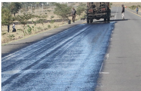
Figure 27. Application of binder for the control section.
