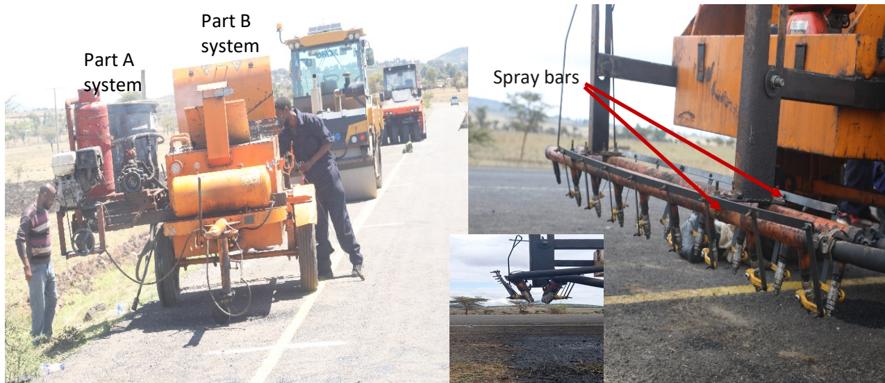
Figure 25. Set up of the MECS plant and the spray bars.
