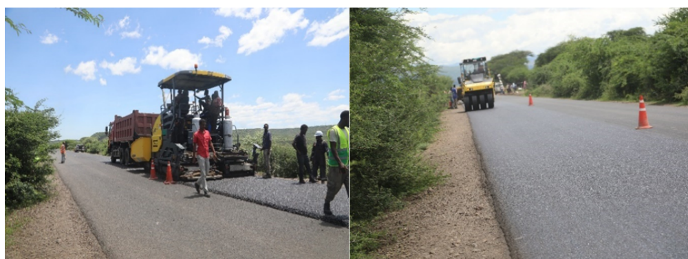
Figure 31. Construction of FMA surfacing
