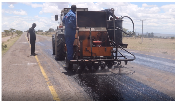
Figure 26. Epoxy binder application for MECS
