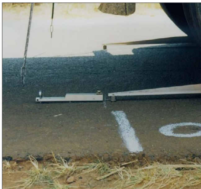
Figure 11-2: The Dehlen Curvature Meter
