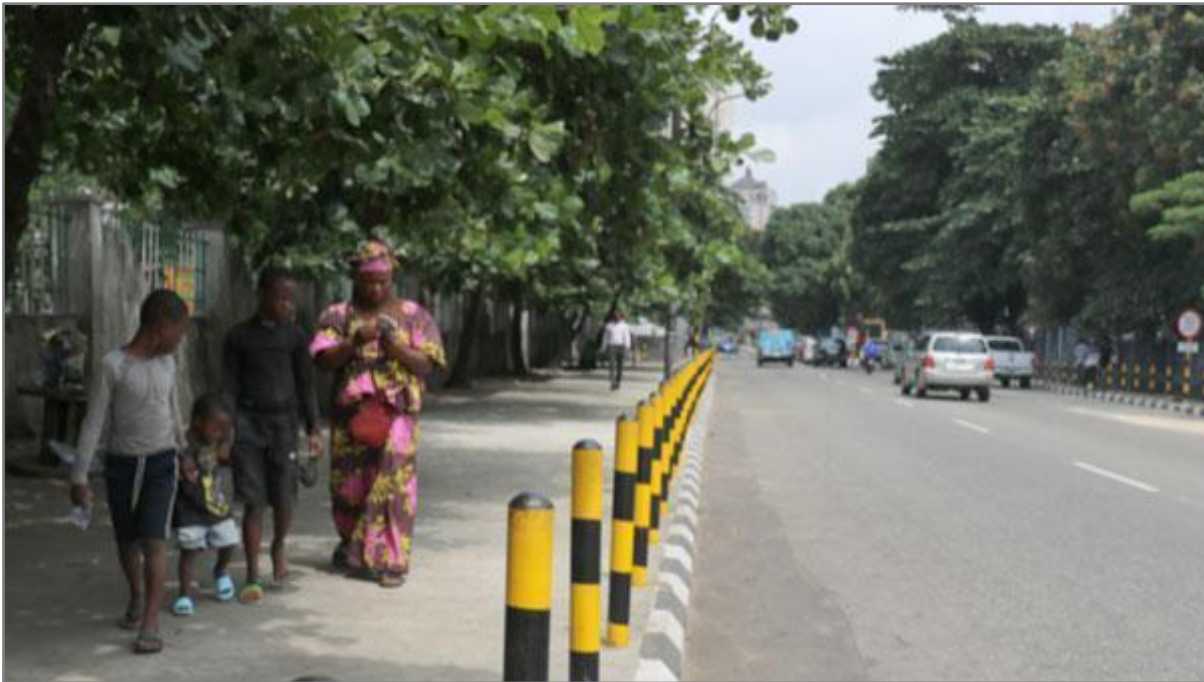
Figure 5: Footpath AFTER upgrade by LAMATA
