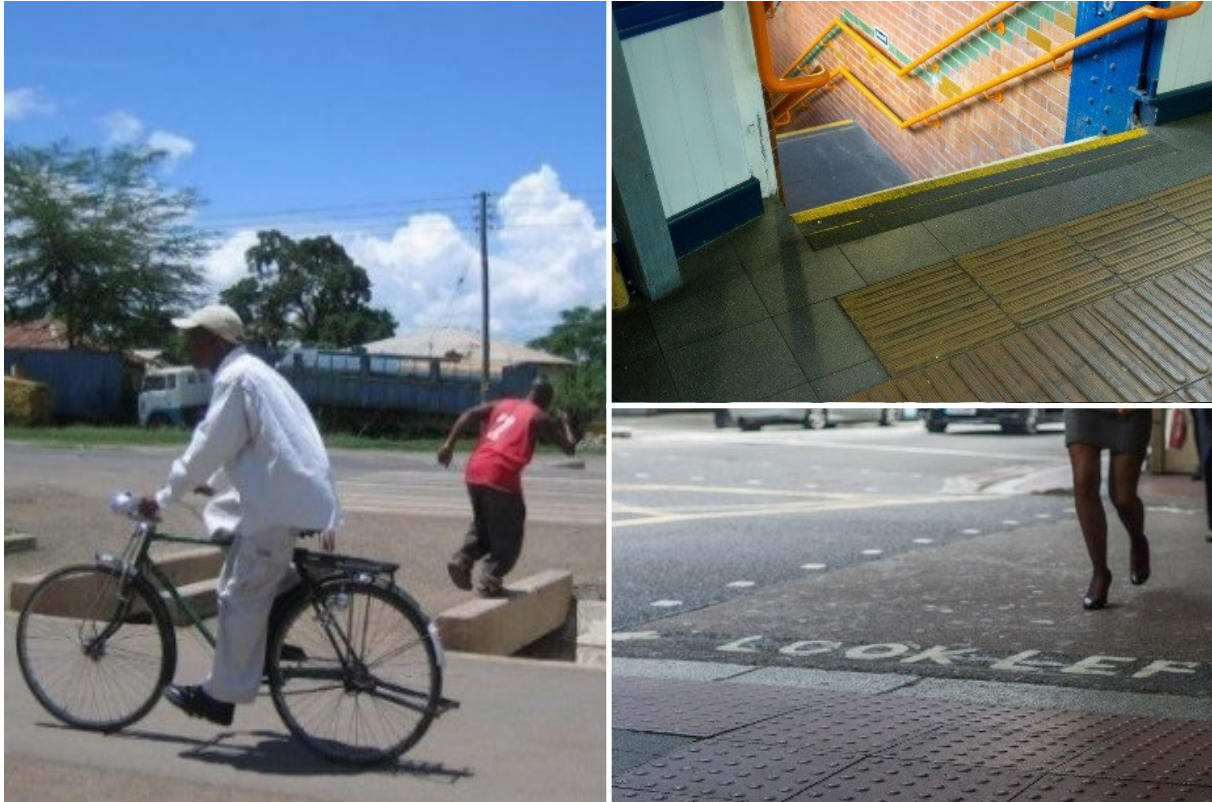
Caption (From left, clockwise): In Tanzania, a level crossing of a drain creates access for wheelchair users, but without warning signals, the crossing is potentially dangerous for people with impaired vision. Photo: Access Exchange International. Photo 2 (top right). London, UK, a warning surface at the top of stairs. Photo 3 (bottom right) London, UK, guidance/warning surface used in conjunction with a flush dropped kerb at a street crossing. Photos: John Frye Photography
