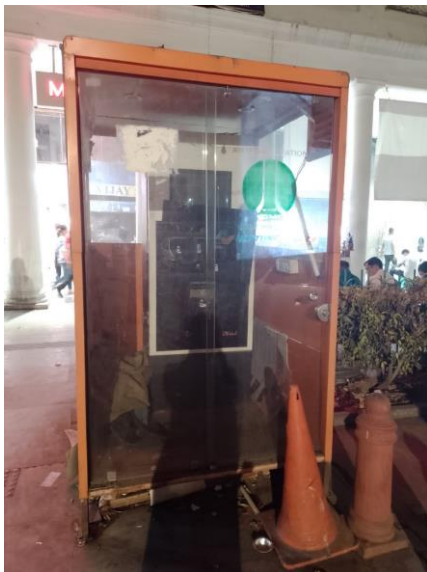
Figure 40: Charging point covered with a protective box to prevent vandalism (Rajiv Chowk)
