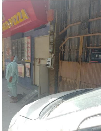
Figure 39: Charging point positioned amidst electricity meters
