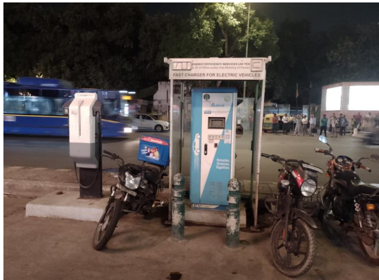
Figure 41: Charging gun and digital screen missing due to vandalism (Rajiv Chowk)
