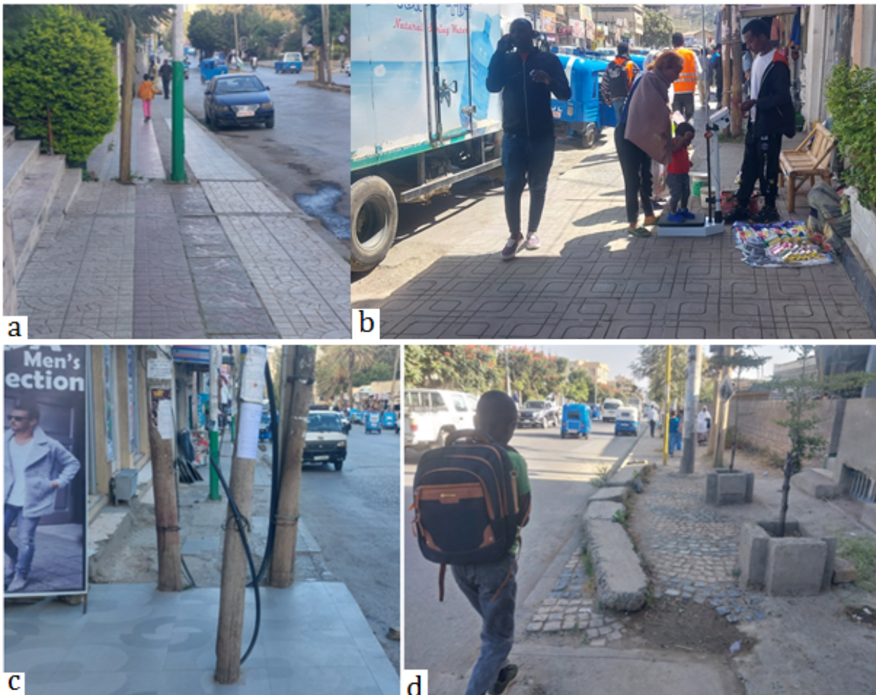
Figure 3-11: Sidewalk obstructions in Mekelle city main streets: Alula Street (a, b, c) and Adihawsi-Hawelti Dldi Street (d)
