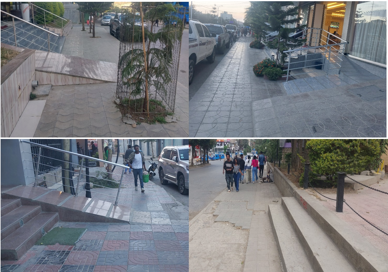
Figure 3-16: Access ramps and stairs in some public/commercial buildings extended onto street sidewalks in Mekelle city
