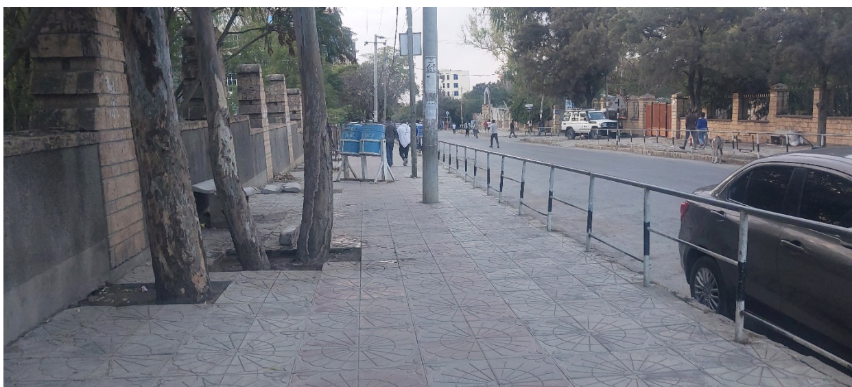
Figure 3-13: Poor sidewalk space management on the Agazi Street in Mekelle city
