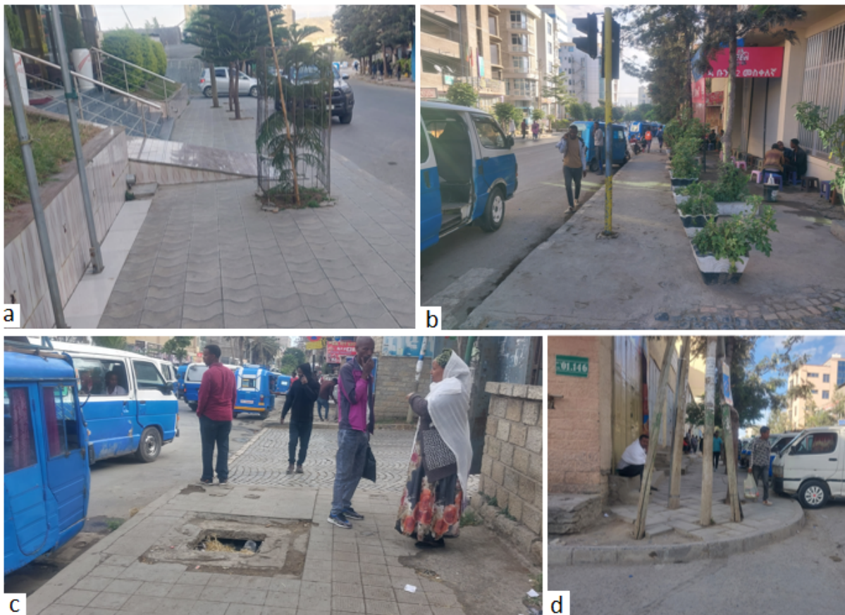
Figure 3-12: Obstacles and safety hazards on sidewalks of Mekelle city: extended ramp and tree with planter box (a); sidewalk café, planter container and street furniture (b); open manhole (c); and missed ramp, congested utility poles and perpendicular on street parking (d)
