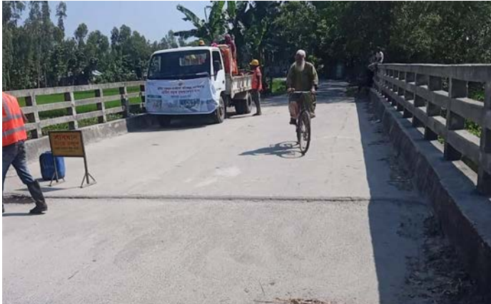
f) Vertical gap between bridge approach and bridge deck will create significant distress for Tri-SMV users
