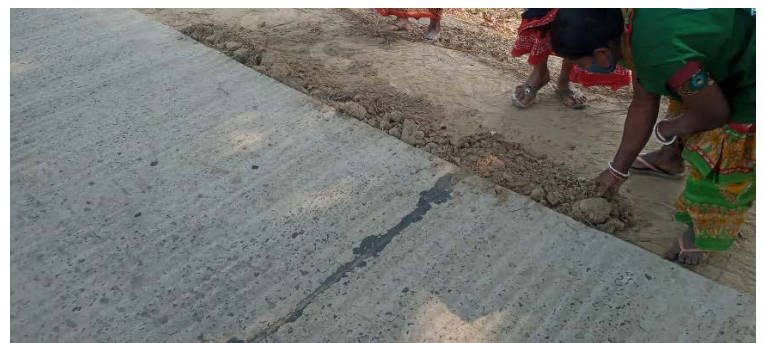
d) Expansion joints as well as rigid pavement texture may result discomfort for Tri-SMV users while steep shoulder drop may result accidents
