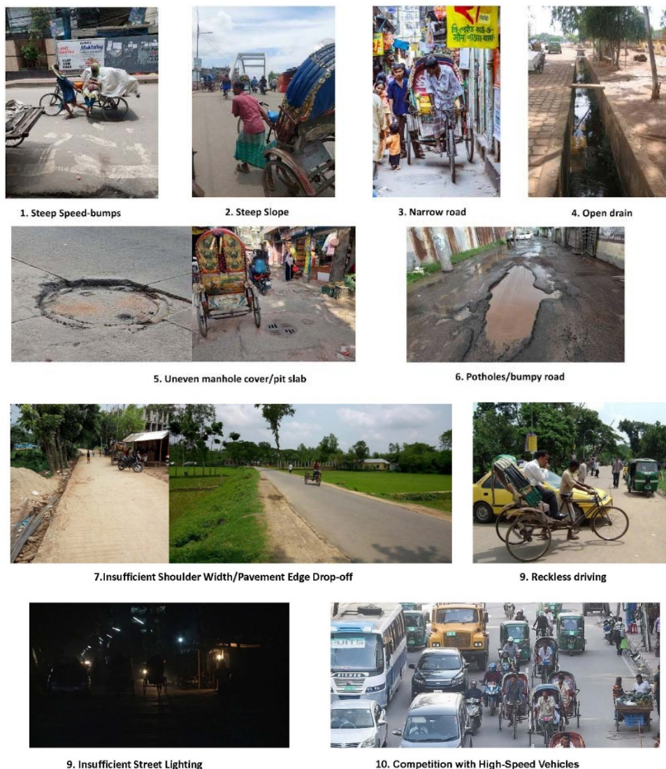
Figure 5 Identified Road Hazard and Discomfort issues.
