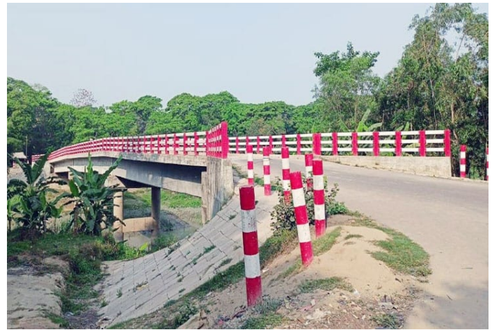
d) Steep approach road may result lack of control; also notice the gap between edge barrier posts and sharp turn
