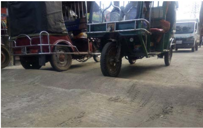
a) Speedbreakers are disproportionate for Tri-SMVs
