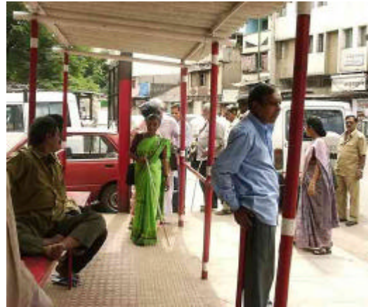
Figure 4: Low-cost interventions to bus stop include use of tactile paving, high contrast paint, and installation of benches.
