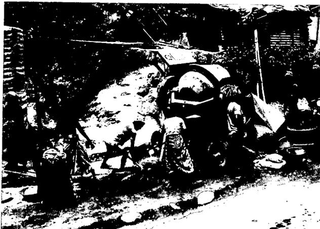
Fig 8 Cement stabilized gravel being mixed and loaded into headpans
