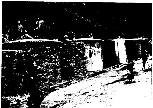
Fig 10 The replacement cylinder wall nearing completion. From left to right the skin types are: two of dry stone masonry, three of galvanised steel sheet (one bitumenised), two of bamboo palisade (one bitumenised), and two without a skin (temporary polythene skin removed after curing). Caps on cylinders are made of mortared stone with a tile eave
