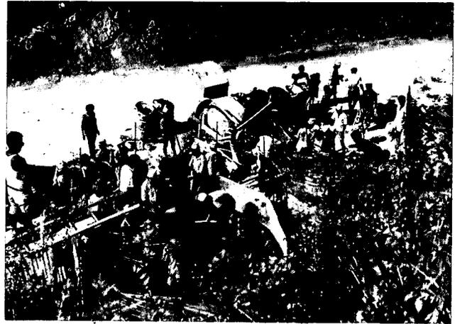
Fig 9 Spreading and tamping cylinder fill material
