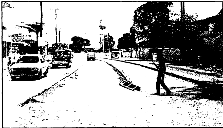
■ Figure 2. Road widening and rehabilitation in Manila.
